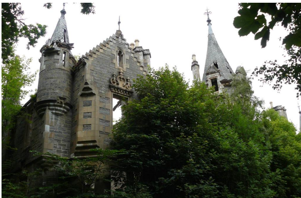
Overgrown ruins of the estate house, Dunalastair, August 2013
